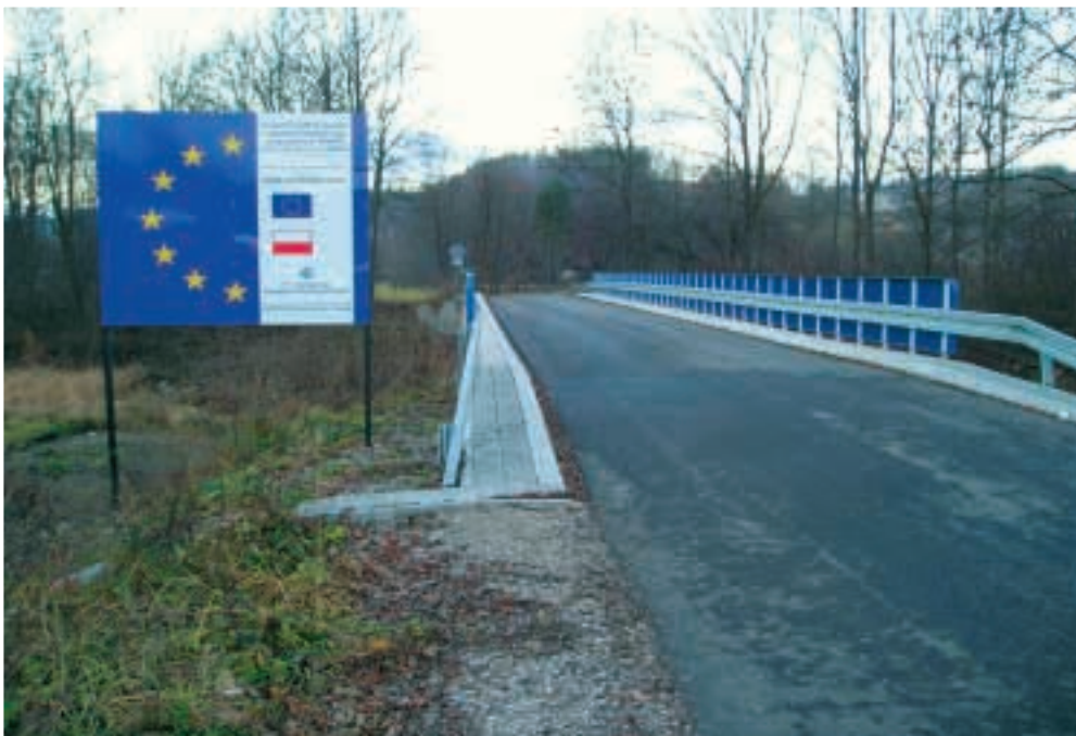
Fot. 3. Widok na odbudowany most Photo 3. View of the reconstructed bridge
