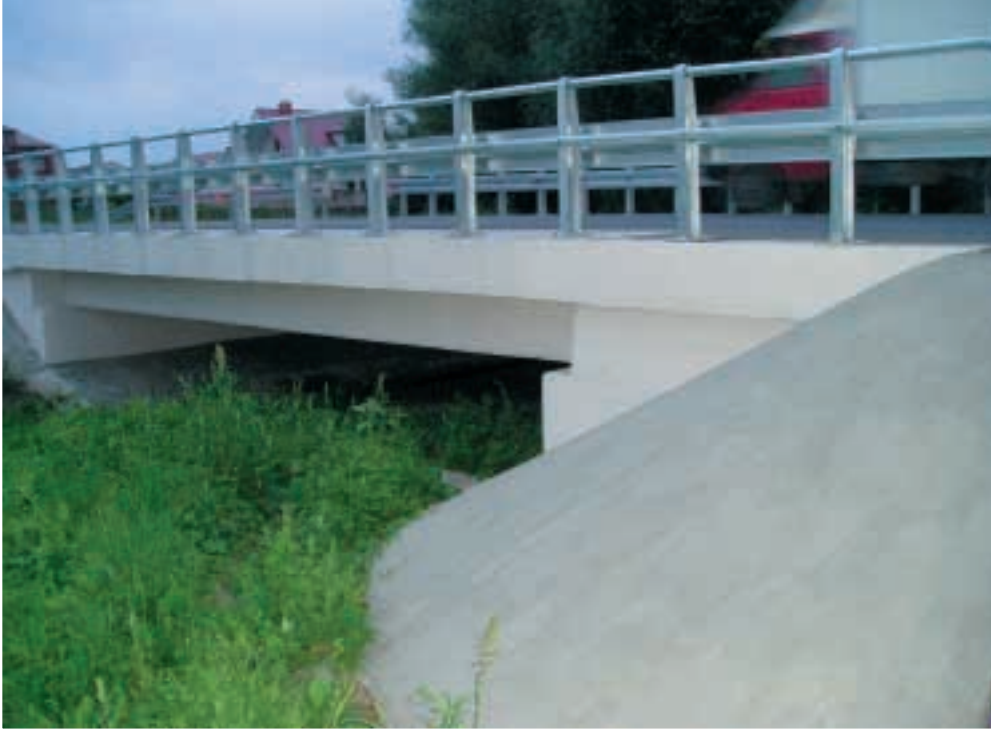
Fot. 32. Widok na odbudowany most Photo 32. View of the repaired bridge
